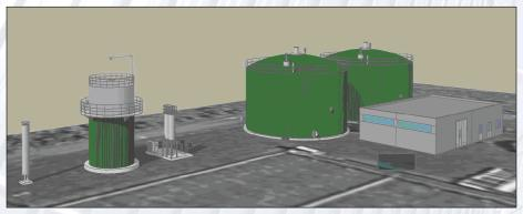
The biogas is transformed in thermic energy in a specific boiler to supply heat for the wastewater treatment plant processes. This solution will allow for the reduction of the energy costs of the whole plant up to 50%.
